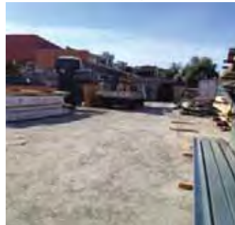
View of: Timber storage yard toward Mitchell Street Looking north
